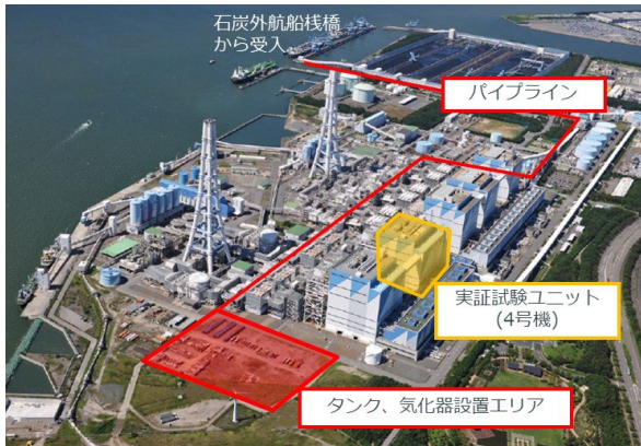
Photo-1 Project 1: JERA Hekinan Thermal Power Station Unit 4
